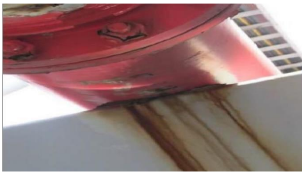
Corroded Pipe
